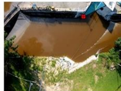
Position 4 [B] Blickrichtung in den Bypass
